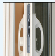
Two-point mortise locking system securely locks the door into the jamb.
